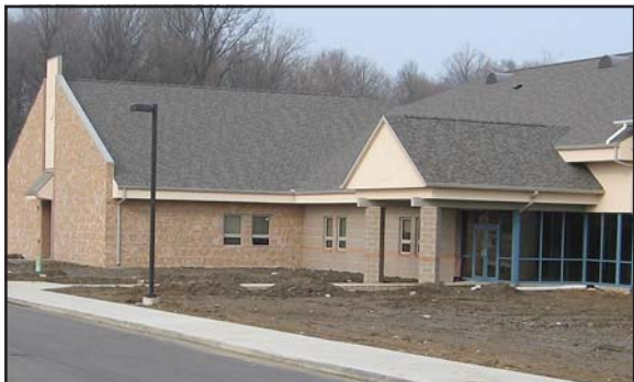
Phase I of a $4.2 million school expansion at Bashor Children's Home is complete. Next up is a new 250-seat dining room and new food services facilities. The entire 34,000 square foot project should be completed by September.
