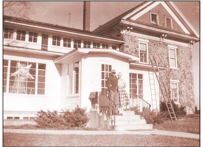
The original Bashor family farmhouse provided care for orphans and troubled boys from 1923 through 1987. John and Emaline Bashor donated 160 acres of land west of Goshen to The Methodist Episcopal Church for the expressed purpose of caring for children.
